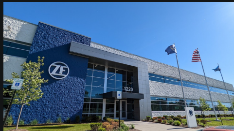
Figure 1: Source: google.com ZF Group Office in Auburn Hills, MI
